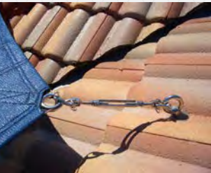
Photo: An installed rafter bracket assembly attached to a shade sail
